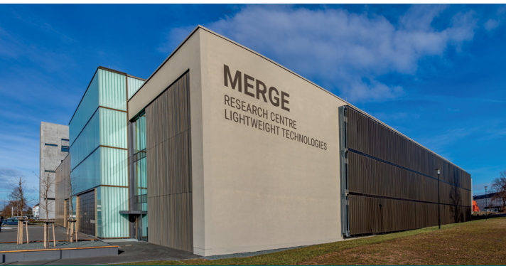
1 The new laboratory building at the MERGE Research Centre Lightweight Technologies is directly adjacent to the MERGE research hall already completed in 2015.
